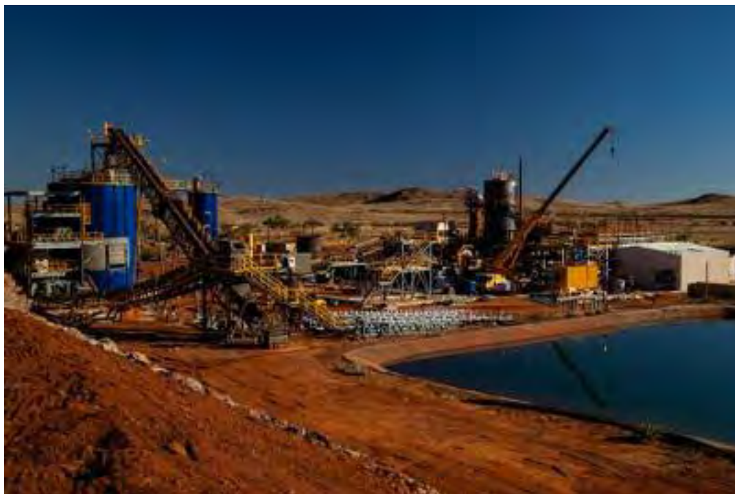
Figure 29: Radio Hill plant
